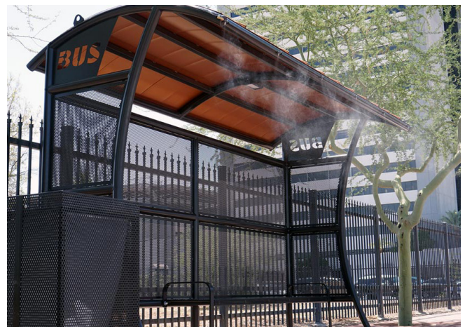
Bus shelter with cooling features
