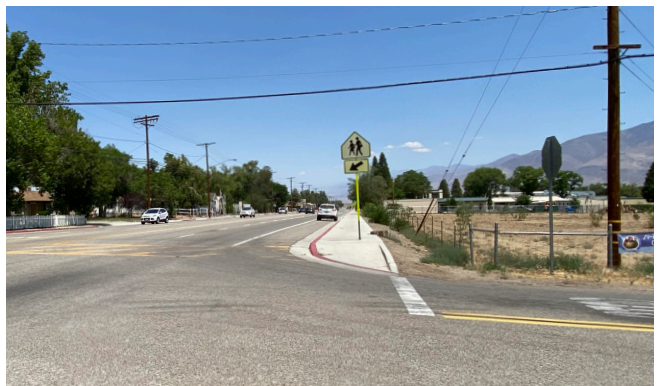
Existing unsignalized crossing at Highway 395 and Bartell Rd
